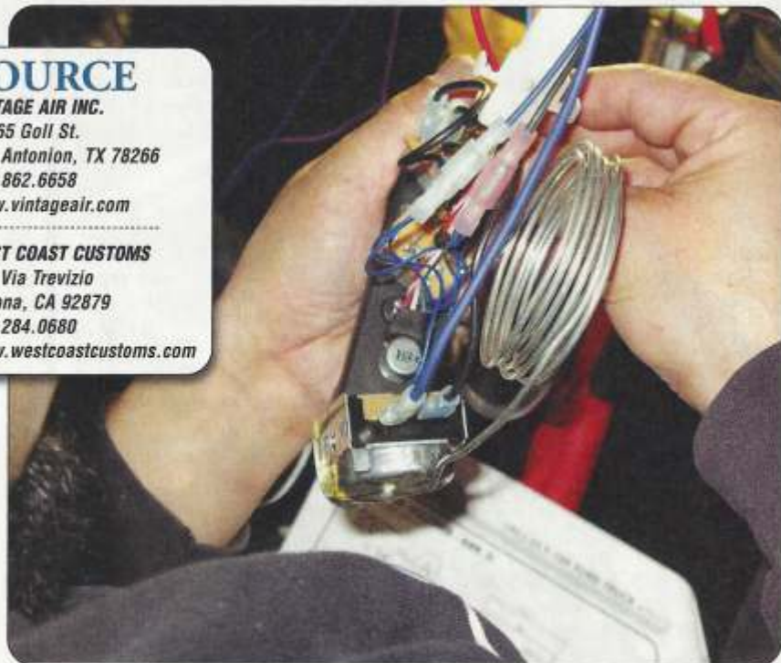
Mosco actually wanted to test the wiring on the controls in a position where he could easily get to it, so he connected all of the wires while the controls were still uninstalled.
