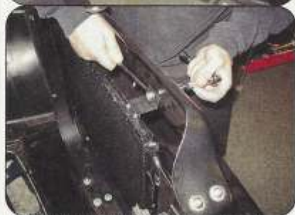
The next item to be installed was the condenser. It actually just bolts onto the factory core support and uses existing holes!
