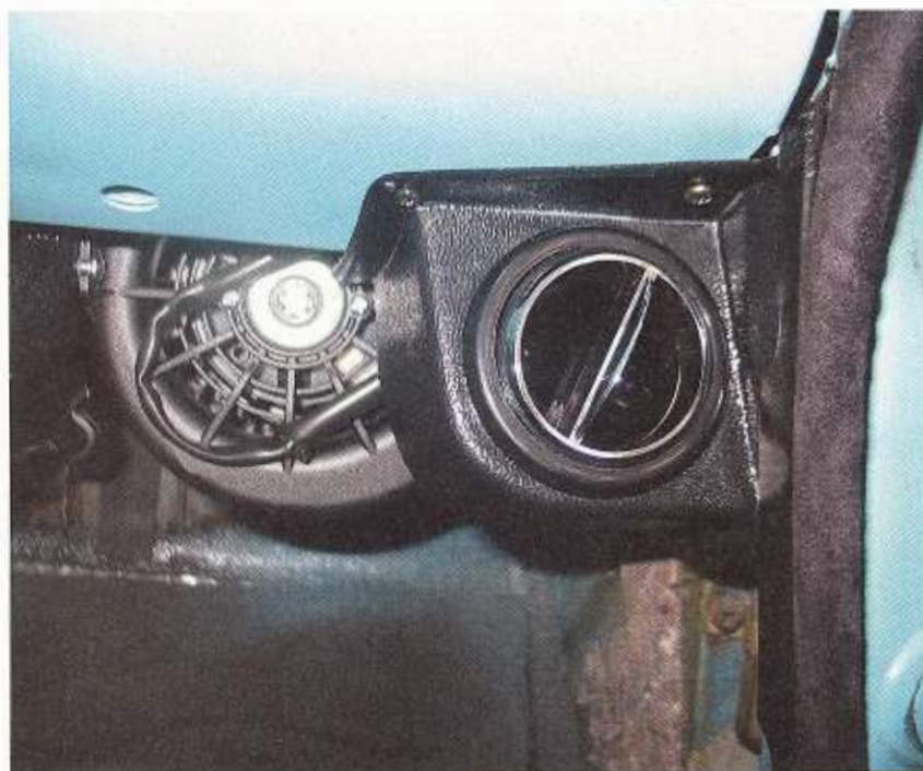
With the side vents in place, you'll run all the ducting to the defrost vent, center vent and two side outlets. Now you're ready to take your system to your local air-conditioning specialist to have your system charged.
